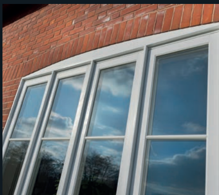
Mullion stiffener used to replicate the original aesthetics of the windows.
