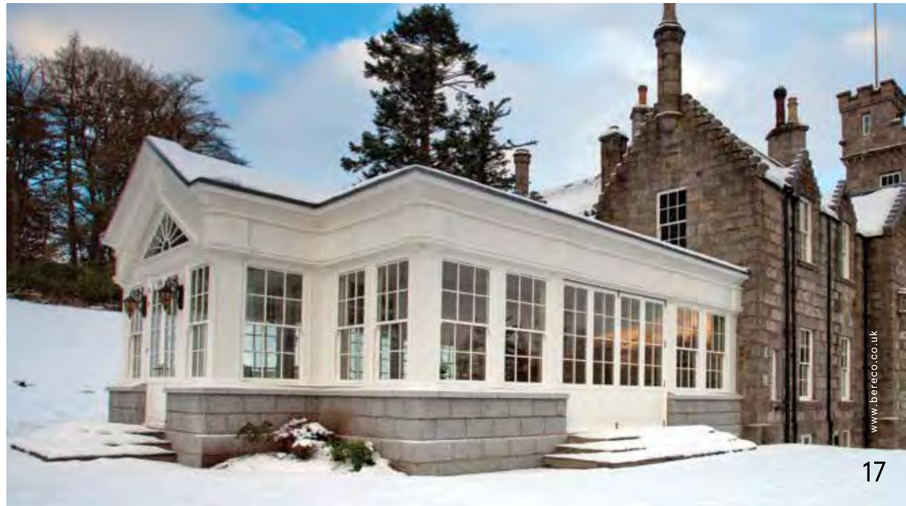
TOP IMAGE shows Heritage Range Sliding Sash Cords & Weights Windows with 25mm Georgian bar design and 14mm SlimLine double glazing. Finish is RAL 9016 Traffic White.
